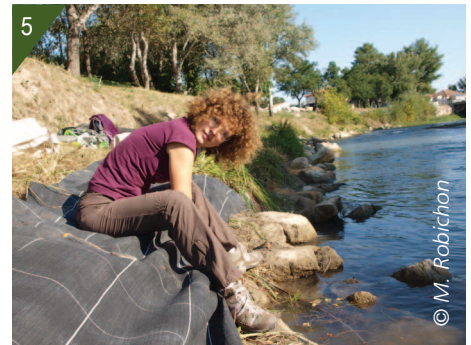
5. Installing the tarp.
