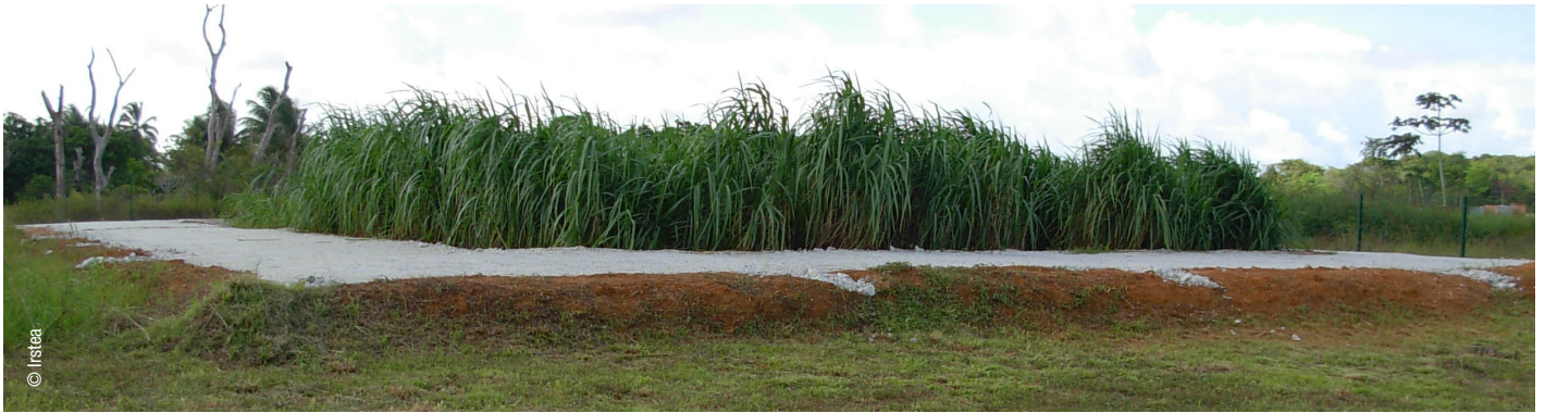
Irstea is working on adapting sophisticated water-treatment techniques to the overseas context. The photo shows a planted filter (reeds) at a wastewater-treatment plant in Macouria (Guiana).
