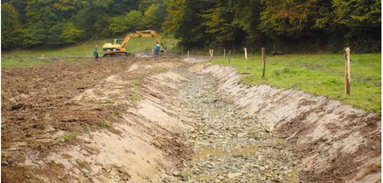
The works phase during the restoration of the Doquette in October 2008: introduction of coarse materials in order to reconstitute the alluvial mattress of the river bed.
