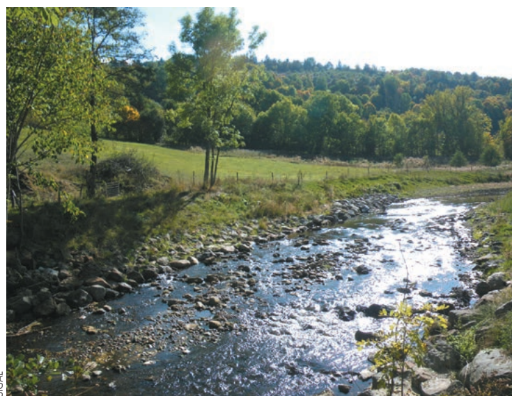
View after removal of the weir in November 2009, the vegetation has partially grown back and the river bed is more diverse.
