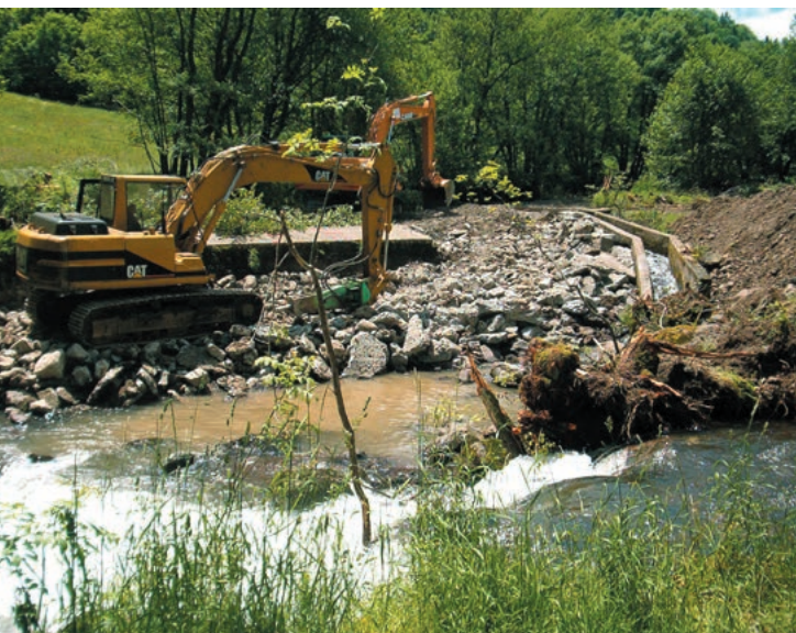
Removal of the Stalapos weir during the excavation phase of the project in June 2008. The river was diverted to dewater the weir and the impounded reach.
