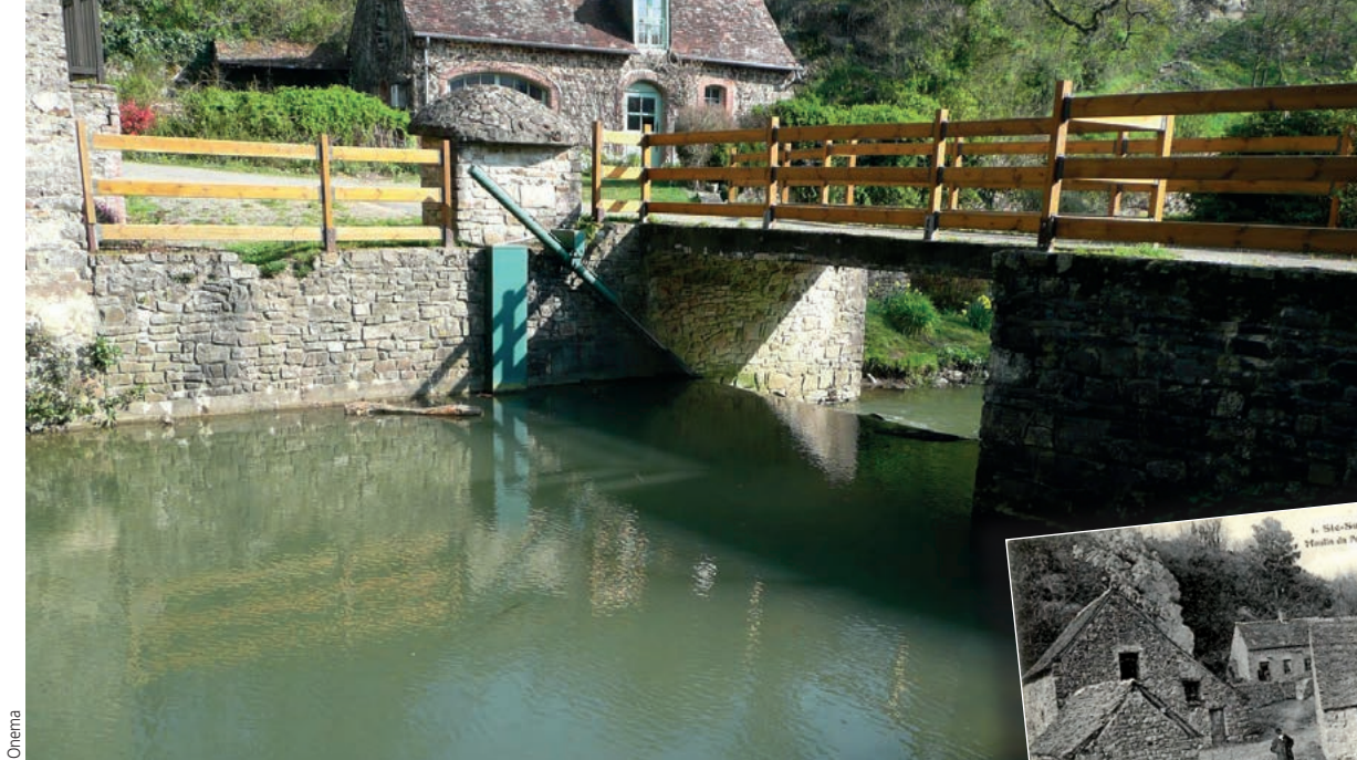
The Grand-Moulin (Great Mill) prior to removal of the flap gate.
