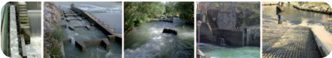
1- Baffle fish pass. 2. Pass with consecutive basins. 3. "Natural" pass. 4. Fish lift. 5. Device specifically for eels on their spawning runs, allowing them to "crawl" between the studs
