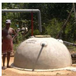
**Figure 47 :** Cuve semi-enterrée (dome tank) (source : T. Thomas)
