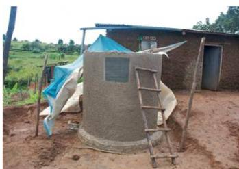
**Figure 45 :** Cuve en ciment (ferrocement tank) (source : Kigezi Diocese WSP)
