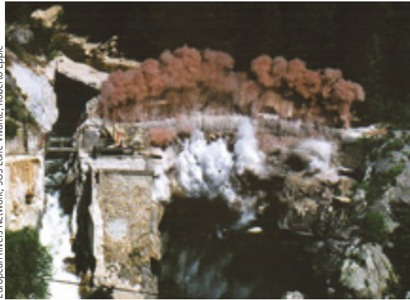
The demolition of the Saint-Étienne-du-Vigan dam in June 1998, using dynamite. The river water was rerouted along the right bank.
