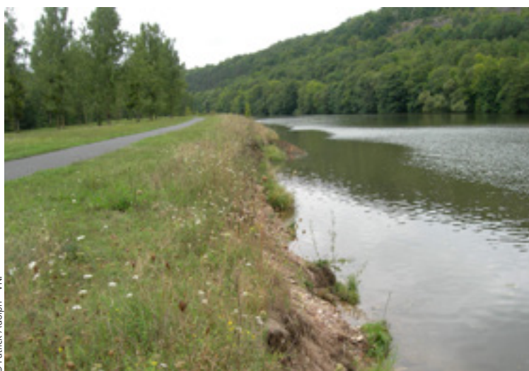
Eroded sections appeared in the banks following the collapse of metal sheet piles along the Moselle River. August 2008.
