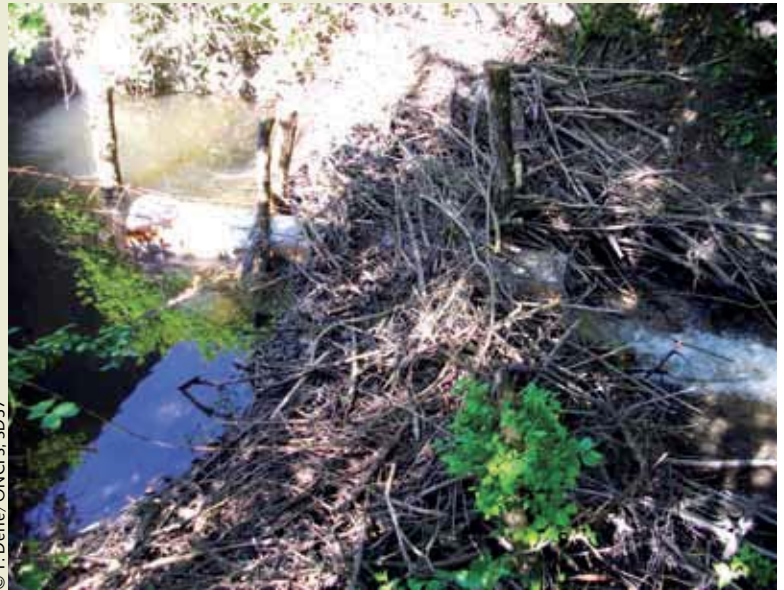
© F. Derré/ONCFS, SD37
