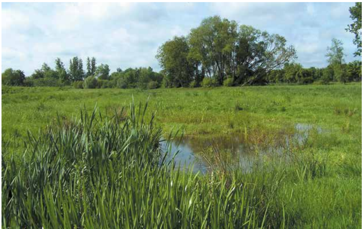
Flood plain of the Vezouze. Flood channel on the left bank - 2 years after the work - May 2009
