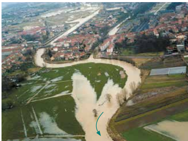
The Vezouze at Lunéville before restoration work. The levee on the left bank prevents flood storage in the flood plain
