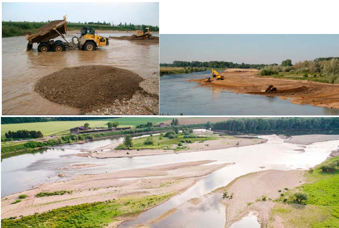
Figure 5. Gravel augmentation, lowering of banks and gravel pit recovering on the Flemish area in 2009 (Source: maasinbeeld.nl).
