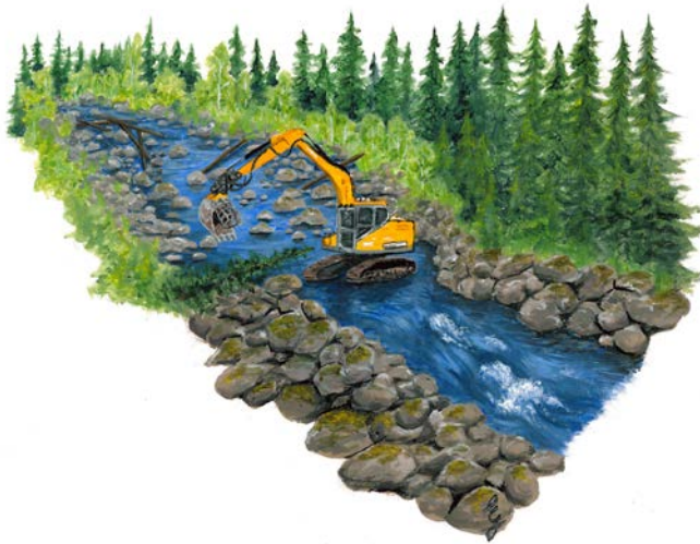
Figure 5. Returning blocks to the riverbed. Source: Ecostreams for LIFE
