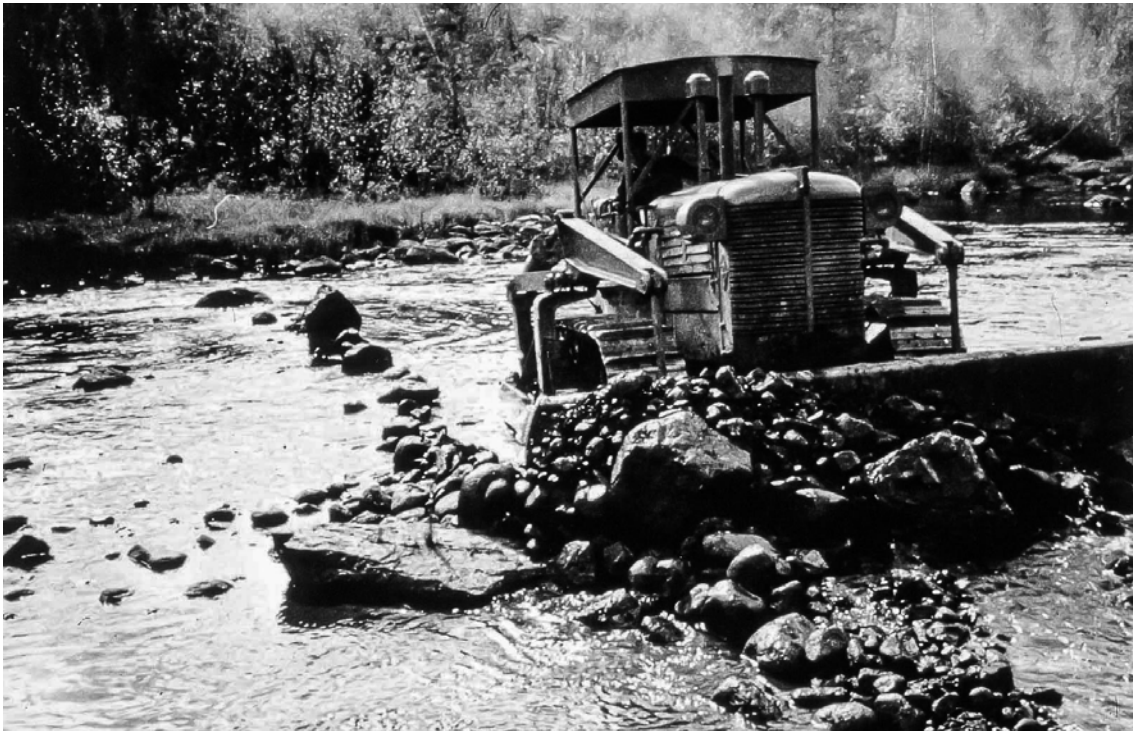
Figure 3. Works of clearance of boulders from the riverbed for timber floating
