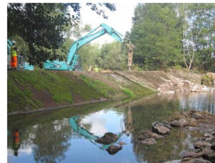
© Natural Resources Wales Demolition of the remainder of the weir continued once the upstream impoundment had been de-watered – 2011
