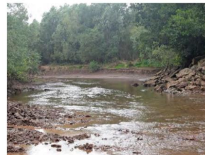
© Natural Resources Wales Looking upstream with the weir completely demolished. The drop in water level is evident on the left bank – 2011
