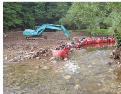
© Natural Resources Wales Line of jumbo sandbags channelling the flow through the initial breach allowing the remainder of the weir and material built up behind it to be removed – 2011
