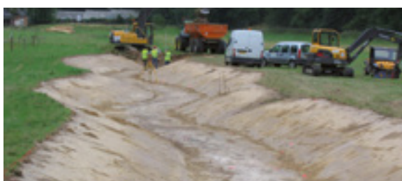
Reopening of the former bed and slight remeandering; Summer 2010
